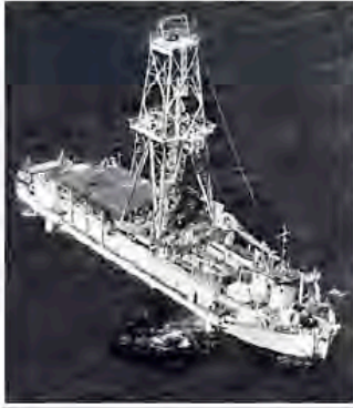
Overhead view of CUSS I, the converted Navy barge used for Project Mohole's deep-sea drilling tests in spring of 1961 (NSF photograph).
