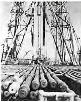
Part of the 13,500 feet of specially-manufactured drill pipe, shown racked in 60-foot double lengths on deck of CUSS I (NSF photograph).
