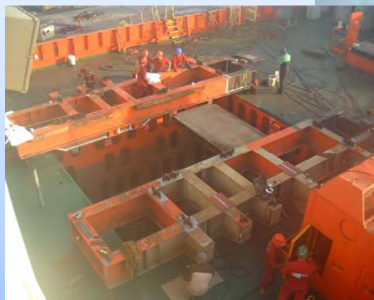
Installing drill rig template
